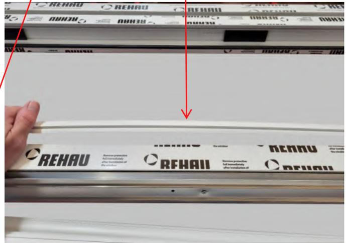
Once each corner of the bead is in place it will require a small amount of pressure to straighten the bead and again tap into place with the rubber hammer into the bead chamber.
