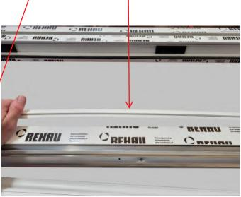
Once each corner of the bead is in place it will require a small amount of pressure to straighten the bead and again tap into place with the rubber hammer into the bead chamber.
